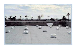
Dark warehouses and commercial office buildings are no match for Natural Light's tubular skylights. Installed on virtually any type of roof surface in under two hours, our 21" commercial units are capable of delivering up to 1400 watts of light without the heat gain or loss of standard framed-in skylights.
